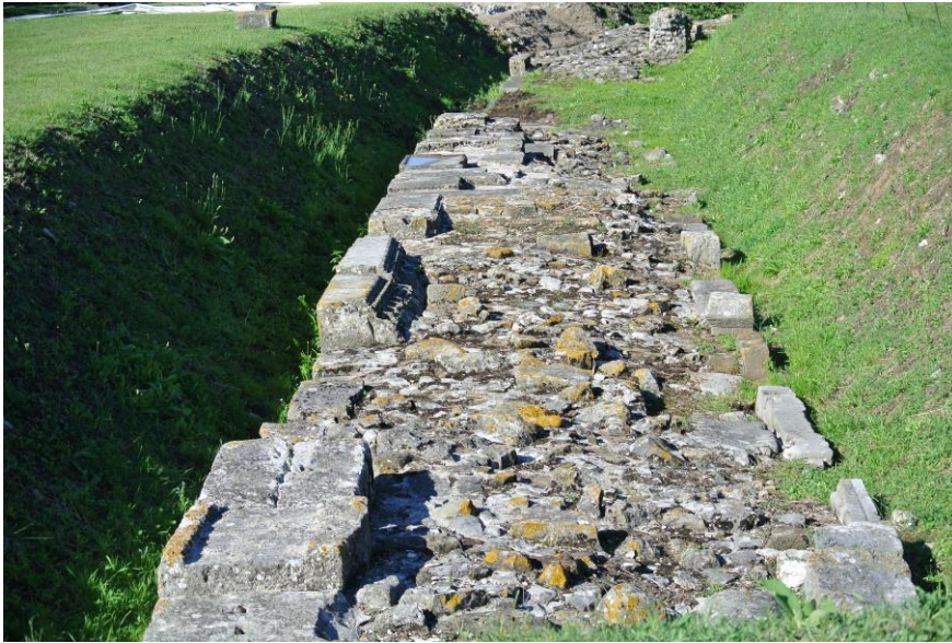
Fig. 10. The inner wall built using recovered materials (bases of statues with inscriptions and parts of moulded cornices) (photograph Patrizia Basso).
