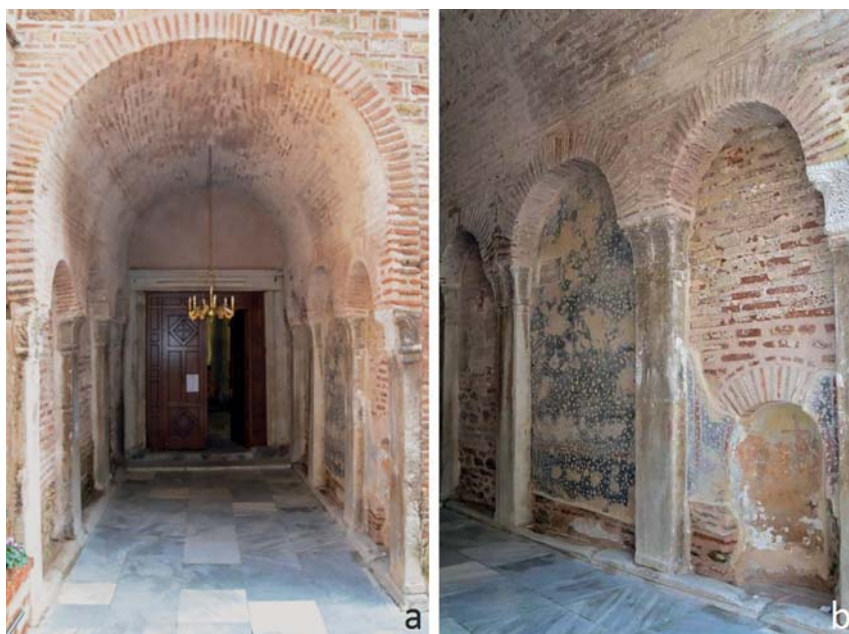
Fig. 2 - Thessaloniki, Acheiropoietos basilica: a) the meridional vaulted propylon; b) the marble pilasters and the east blind arcade of the meridional propylon (photo Konstantinos T. Raptis).
