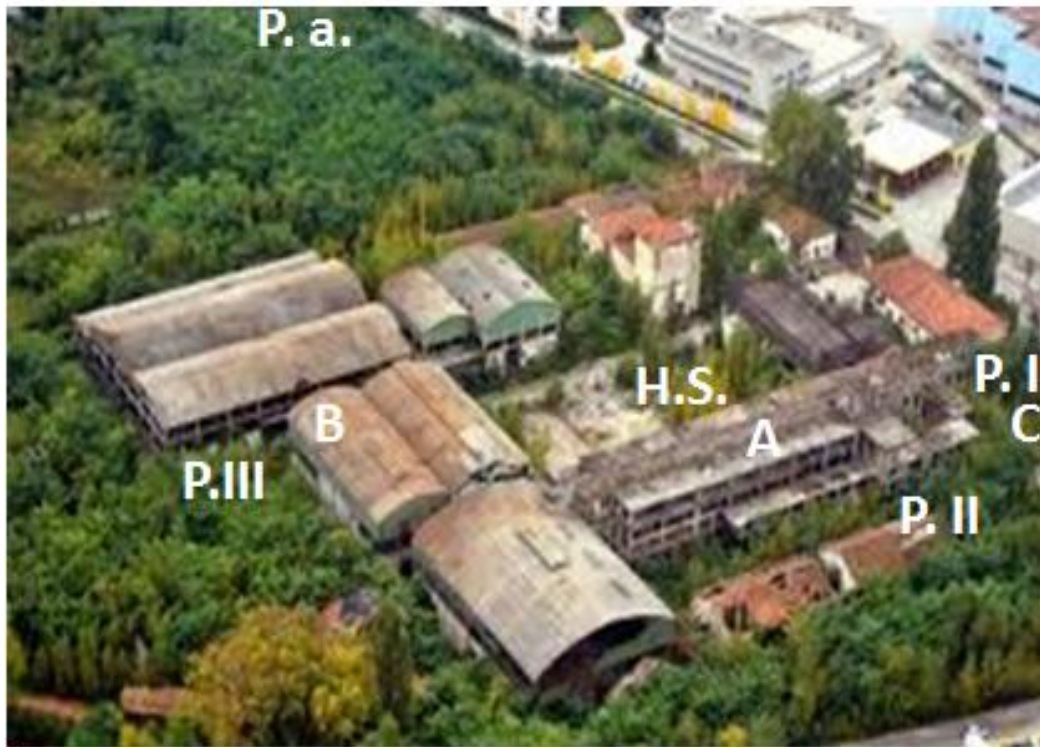
Fig 2.4 Indicative position of the reference points (Point I: P.I, Point II: P.II, Point III:P.III and Hot Spot:H.S), the parking area (P.a.) and of the Reacor section (A), C 2 H 5 Cl production section (B) and Mixer section (C) within the Ex-SLOI area
