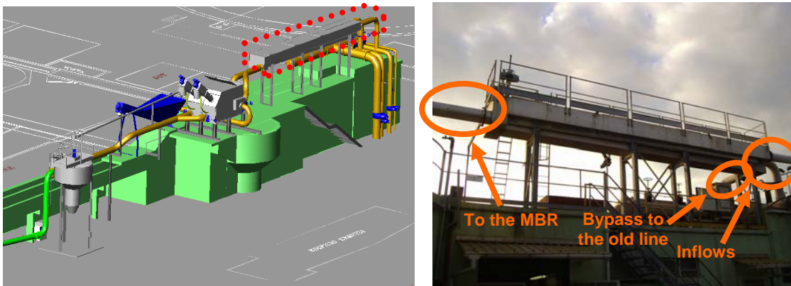
Figure 8.5a-b Drawing (a) and picture (b) of the systems to select the right flow to the MBR
