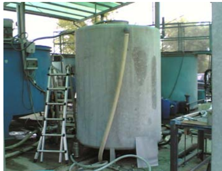
Figure 2.4. Tank to stock the external carbon source
