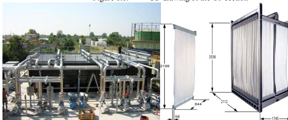
Figure 8.9 a-b-c. Picture of the UF section (a) Zenon membrane module (b) and cassette (c)
