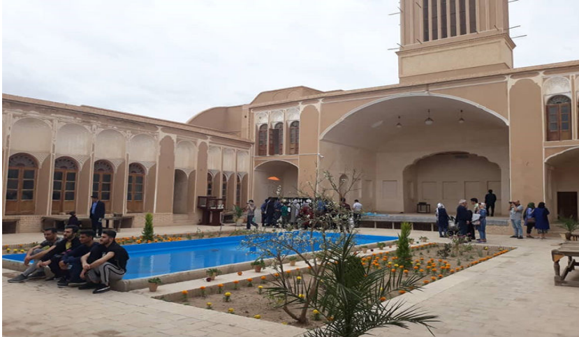
Image 5.10 Yazd Creative House (Heyrani House), Yazd, Iran Source: irancreativehouse.com, (7 June 2019)
