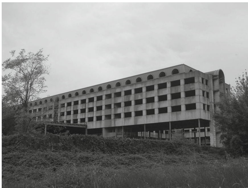
Fig. 15 Abandoned horizontal megastructure, Milan 1972, demolished in the 2000s
