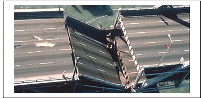
San Francisco-Oakland Bay Bridge Collapse, 1989 Source. Joe Lewis, 2006. https://www.flickr.com/photos/californiawatch/5572600044 [Creative commons license].
